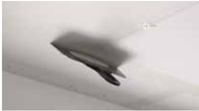
Lay a thin layer of Powder Filler on the joints and fasteners (use 160mm wide knife).
