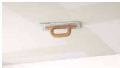
Sand joint down manually.
