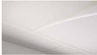
While the Filler is still wet, position the tape on the joints.
