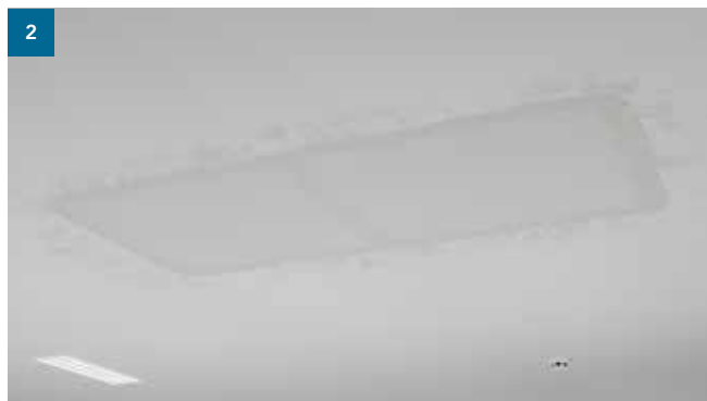
Installing new panels and filling edges. Cut a matching "plug" out of a new Rockfon Mono Acoustic panel and fasten the "plug" in the hole using the filler.
