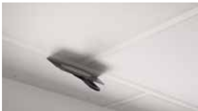
Load the thinned edge with Powder Filler.
