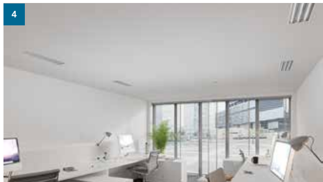
Spraying and removal of masking protections of walls, floor etc. Apply a new layer of the filler on the seam between the "plug" and the panel, following the instructions set out in the guide.
