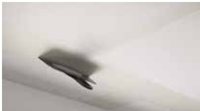
Once the first coat is dry, apply a layer of Ready-Mix Filler (use a 240mm wide knife).
