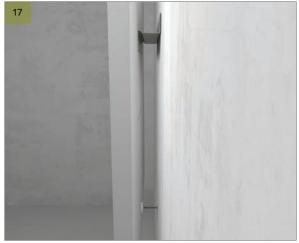
Place your Rockfon® Island™ on the wall bracket and adjust the spacer until the Island is level.
