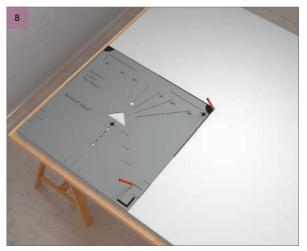
Position the marking tool in the lower left corner on the back side of the Rockfon® Island $^{TM}$ . Mark with a pencil the center lines, using the upper right corner of the marking tool, and the position of the spacer. See 9.
