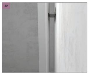
Place your Rockfon® Island™ on the wall bracket and adjust the spacer until the Island is level. See 21.
