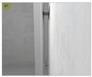
Place your Rockfon® Island $^{TM}$  on the wall bracket and adjust the spacer until the Island is level. See 22.
