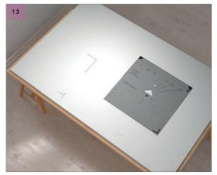
Mark the line where the Rockfon® Island™ Panel Bracket must be inserted. Do this to both the right and left side of the Rockfon® Island™. See 14.
