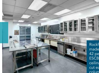
Rockfon's stone wool ceiling panels are made from basalt rock and contain up to 42 percent recycled material to support ESCB's LEED Gold criteria. Stone wool ceiling panels also are lightweight and cut easily to accommodate the facility's columns, light fixtures and sprinklers.
