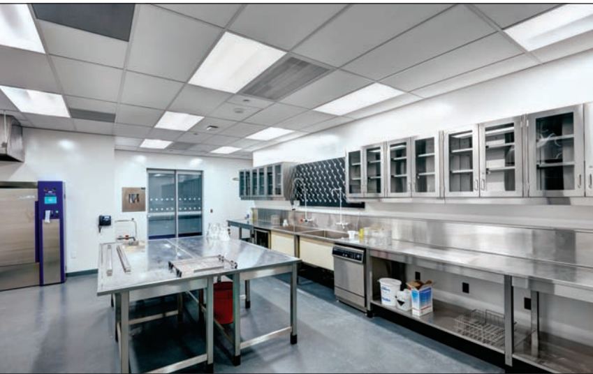
ESCB's laboratories feature stone wool ceiling products selected to meet stringent requirements for air cleanliness in healthcare and cleanroom environments, with finishes that can withstand rigorous cleaning.
