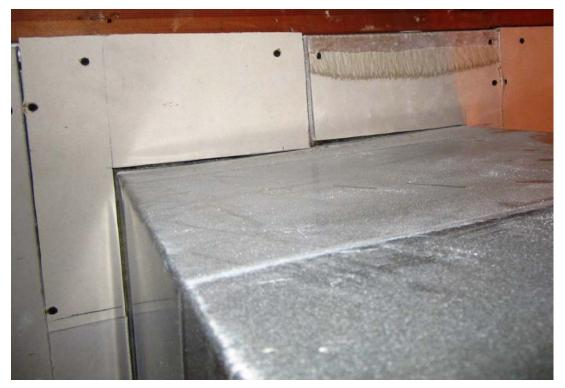
Figure 7: Part of a gypsum board plenum barrier is installed around a supply air duct. The rigidity of the material combined with the imprecise score-and-snap method of cutting the material result in many small gaps and openings.
