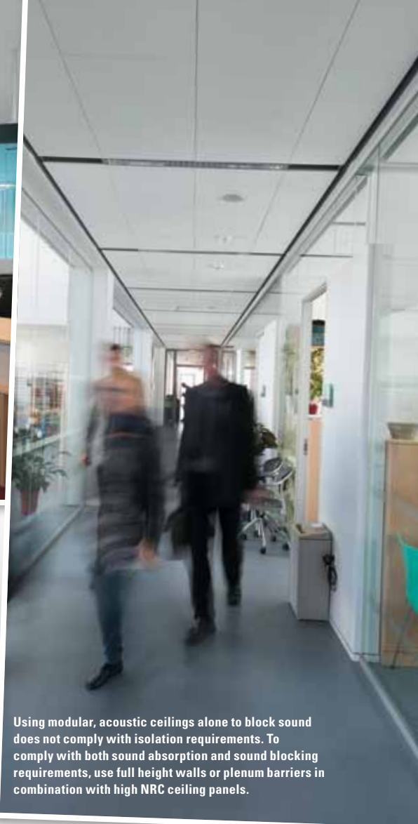
Using high-performance ceiling panels with NRC ratings of at least 0.90 can lead to compliance with the required maximum reverberation times even when there is no other sound-absorbing surfaces in the room.
