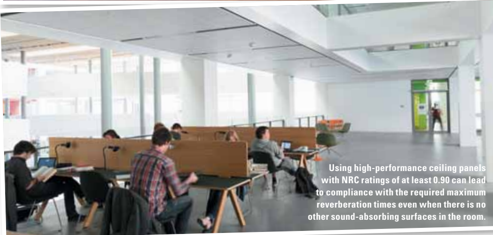
In open spaces, where sound blocking between rooms is not important, using ceiling panels with a NRC rating of 0.90 or higher can lead to compliance with maximum mechanical system and exterior noise levels by absorbing noise that has already entered the room.
