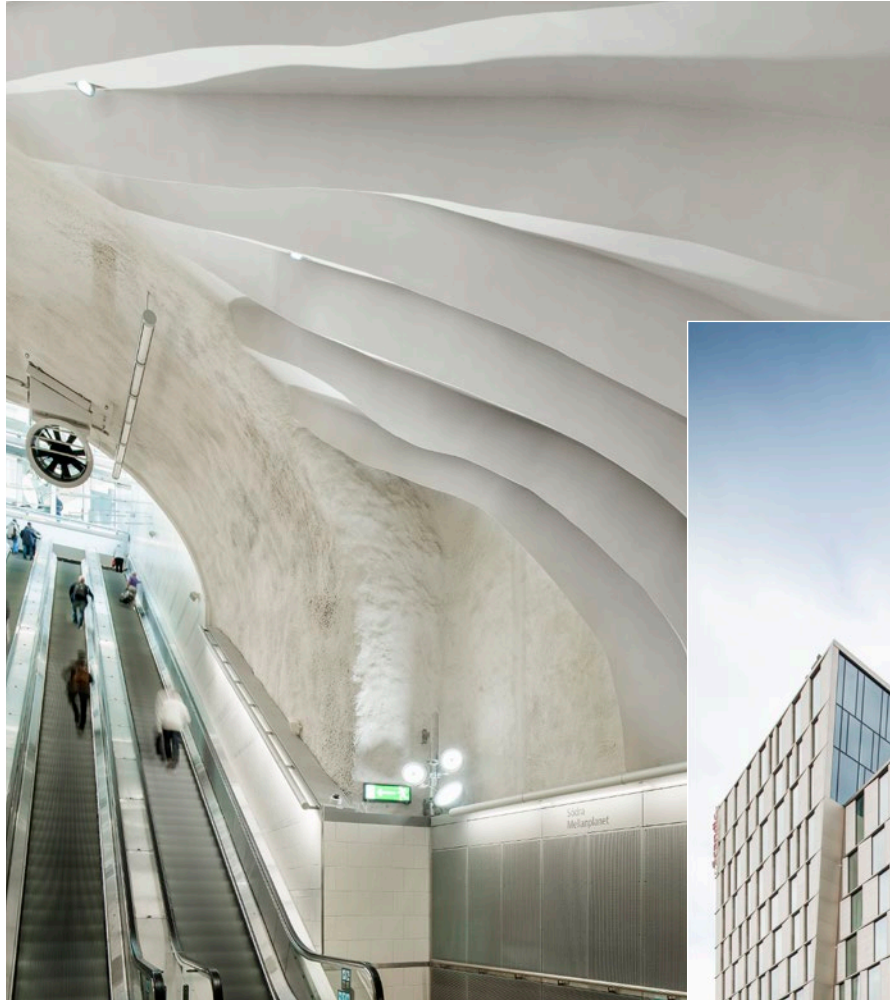
Project Metro station, Stockholm, Sweden Product Rockfon Mono Acoustic white Designer K. Lindh
