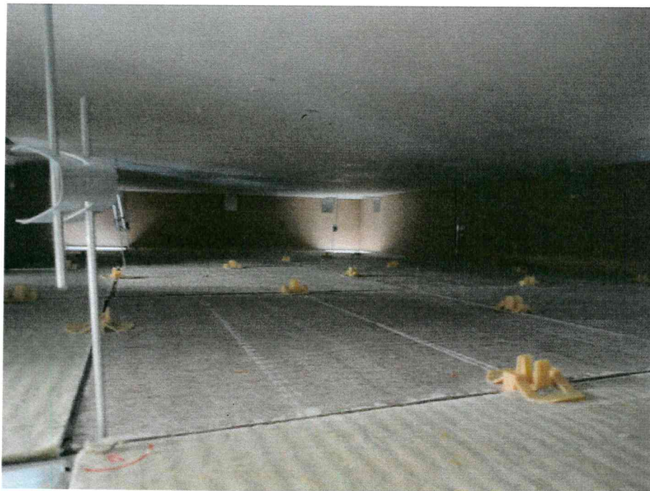
Picture 6: View of the grid system (1200 mm x 600 mm tiles)
