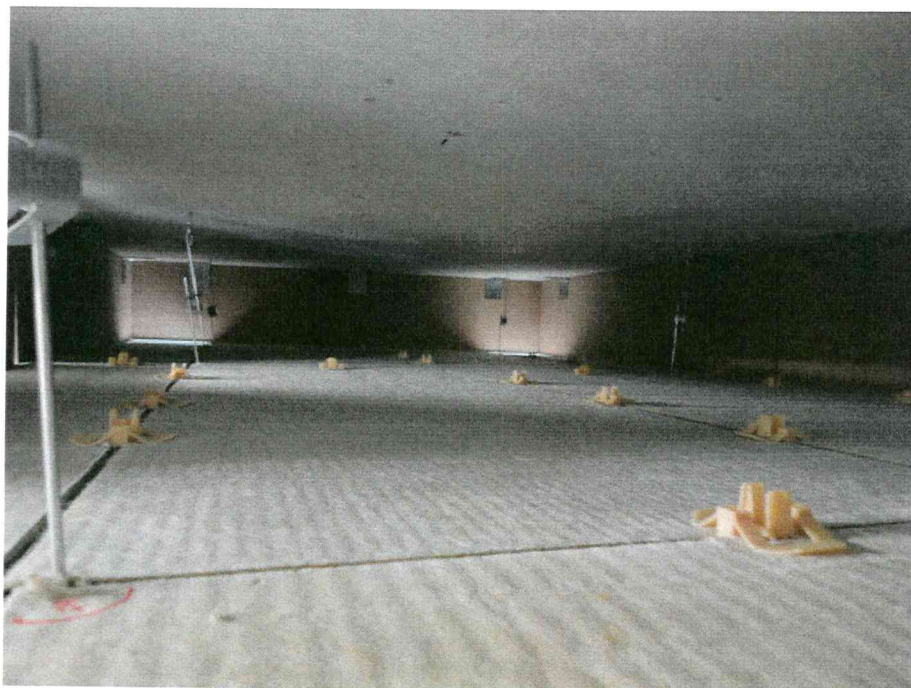
Picture 4: View of the grid system (1200 mm x 600 mm tiles)
