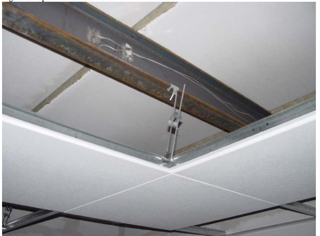
Figure C2 Specimen before the test from the heated side
