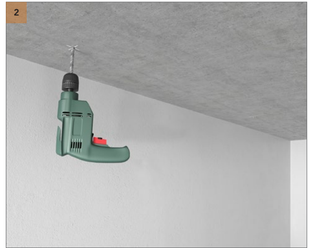
Drill where you have marked drilling points.
