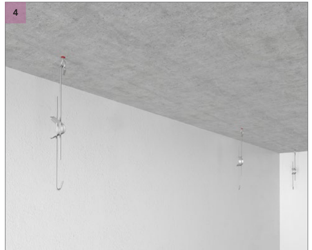
Attach quick-hangers to the screw eyes and remember to secure them by closing the upper hook.
