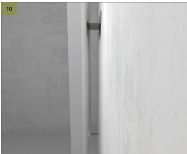
Place your Rockfon Eclipse Wall panel on the wall fixing profile and adjust the distance holder until the Rockfon Eclipse Wall panel is level.
