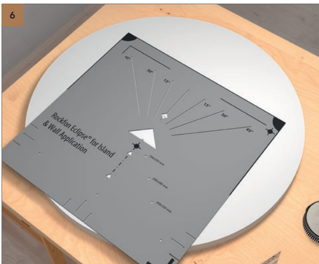
Position the marking tool so that the lines from step 5, drawn around the base of the triangle of the marking tool, are perfectly aligned within the diamond cutout. See 6 - Detail.
