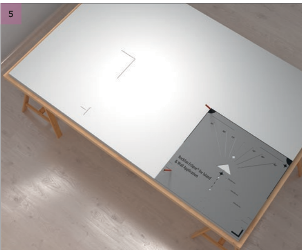
Position the marking tool in the lower right corner on the back side of the Rockfon Eclipse Wall panel. Mark with a pencil the centre lines, using the upper left corner of the marking tool, and the position of the distance holder.
