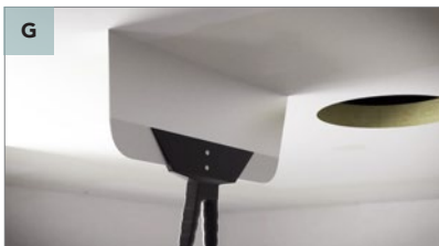
Check joints and centre of panels.
