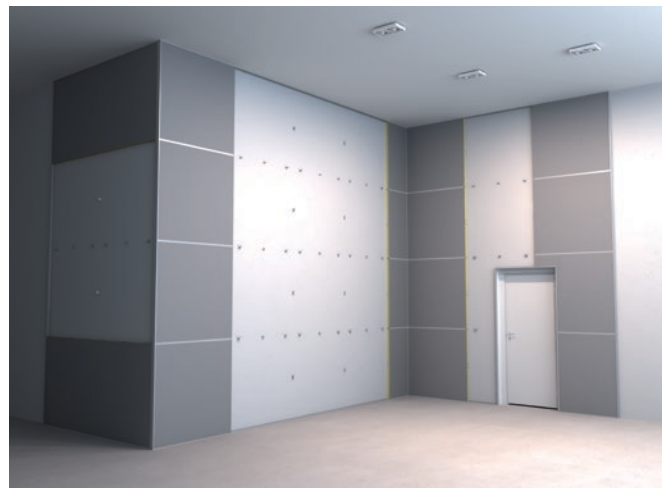
3.10 Cover all remaining horizontal joints between panels by clicking T24 profiles into the T fixing brackets. Horizontal profiles should be cut to an exact dimension of M-12 mm. Ensure the outer ends of the horizontal tees are covered by the J-channels.
