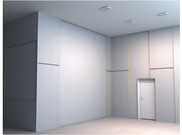
2.3 All outside/perimeter wall panels installed with horizontal HAT profiles.
