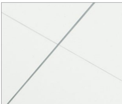
Sharp and straight line created by deeply recessed grid in one direction and a continuous expression in the other direction.
