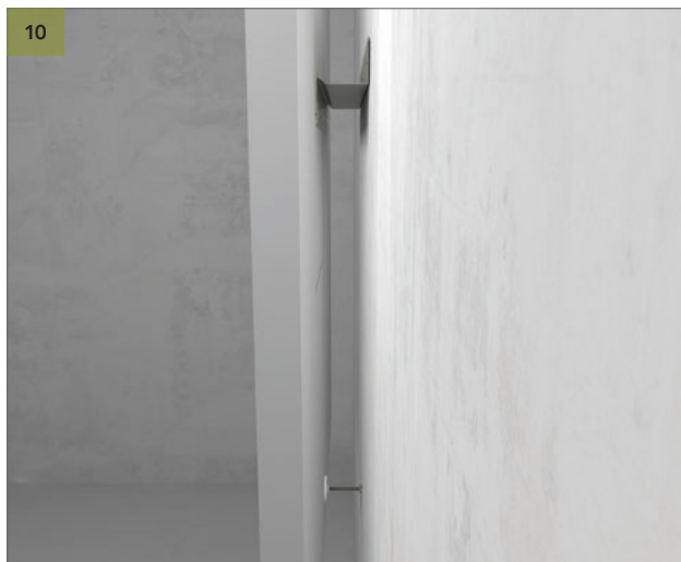
Place your Rockfon Eclipse Wall panel on the wall fixing profile and adjust the distance holder until the Rockfon Eclipse Wall panel is level.
