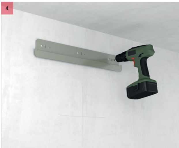
Drill the holes and install the wall fixing profile.
