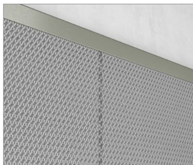
Nice and neat concealed connection between the panels and anodized aluminium perimeter cover profile.
