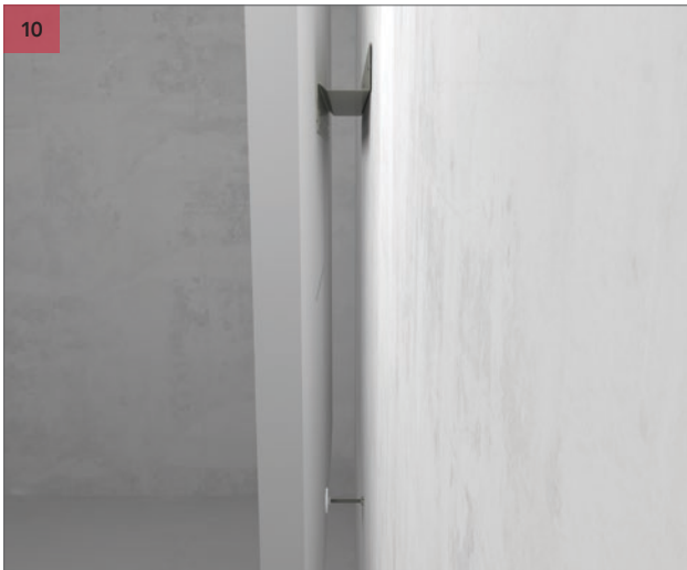
10 Place your Rockfon Eclipse Wall panel on the wall fixing profile and adjust the distance holder until the Rockfon Eclipse Wall panel is level.
