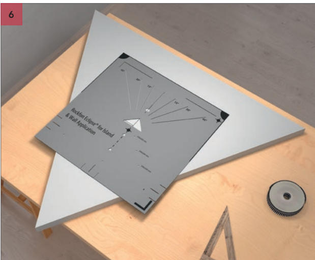
Position the marking tool so that the centre lines drawn in step 5 are perfectly aligned with the point at the base of the triangle on the marking tool. See 6 - Detail.
