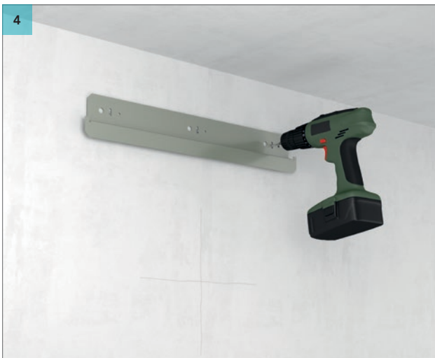
4 Drill the holes and install the wall fixing profile.
