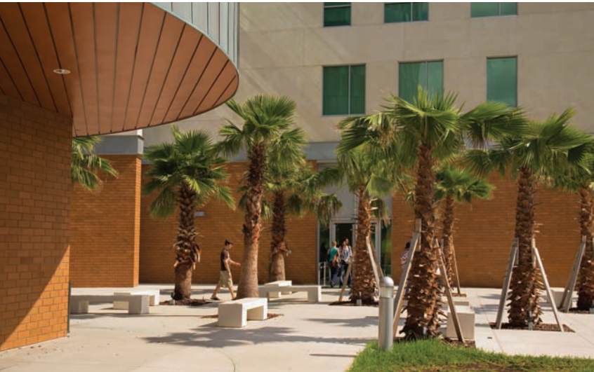
The new Marshall Student Center at the University of South Florida in Tampa features soffits comprising linear metal ceiling assemblies. These are engineered to resist southeastern winds and provide shade from the heat.
