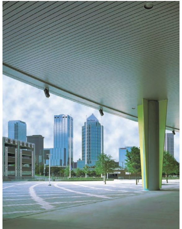
The student center includes materials with completely recycled content such as the soffits' metal systems and suspensions, which typically contain 100 percent post-consumer recycled content.
