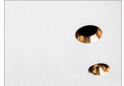
Installed STORM SYSTEM® with flush lighting.
