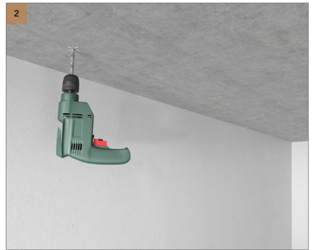
Drill where you have marked drilling points.
