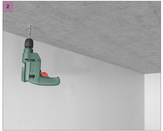
Drill where you have marked drilling points.
