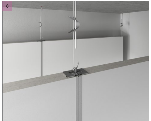
When suspending two Rockfon Industrial Baffles on the same quick-hanger, ensure that the alignment dimples match.
