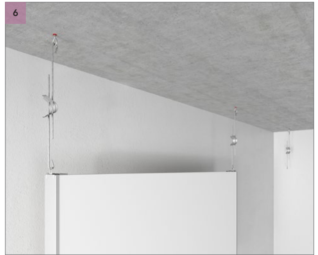
Suspend the Rockfon Industrial Baffles from the quick-hangers.
