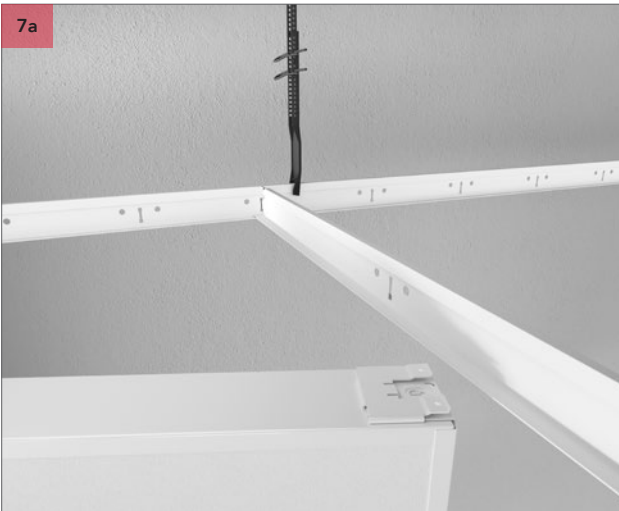
Fix Rockfon Humitec Baffles to the suspended Chicago Metallic T24 ECR grid.
